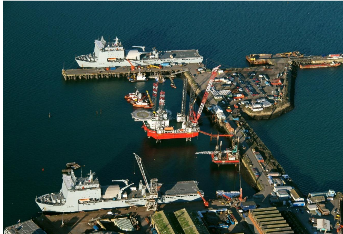
Figure 2: Seajacks Leviathan GI rig docked alongside the location of the proposed FLOW deck
