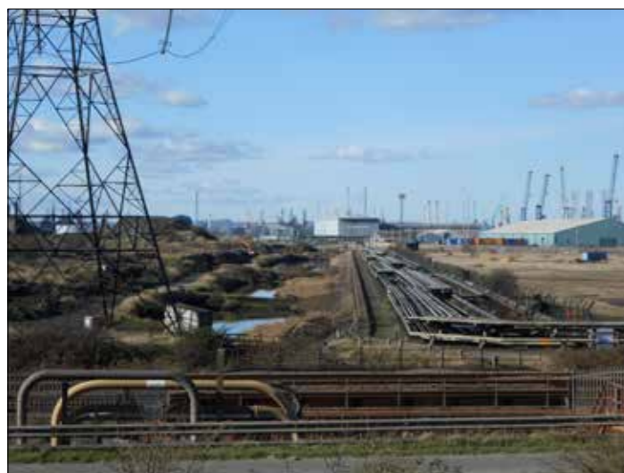
Sembcorp Corridor - West - to No.1 Tunnel
