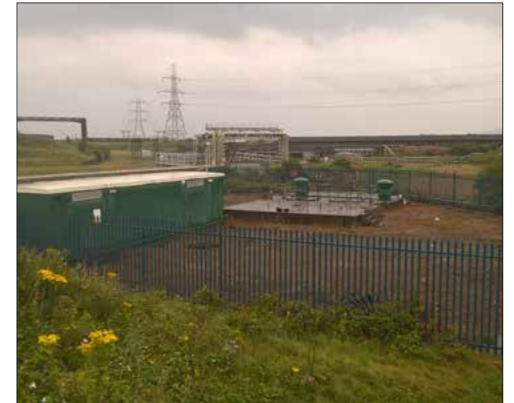
Eston Pumping Station Sewage Transfer Mains
