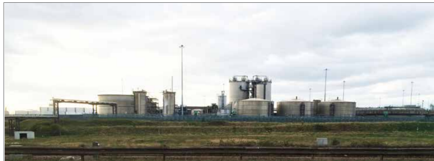
NWL Brand Sands WWTW
