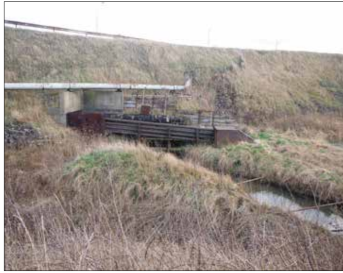
The Fleet - Culvert No.2
