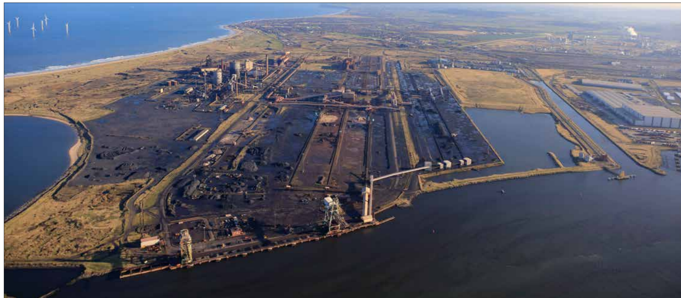
View from the River Tees across the Redcar Site
