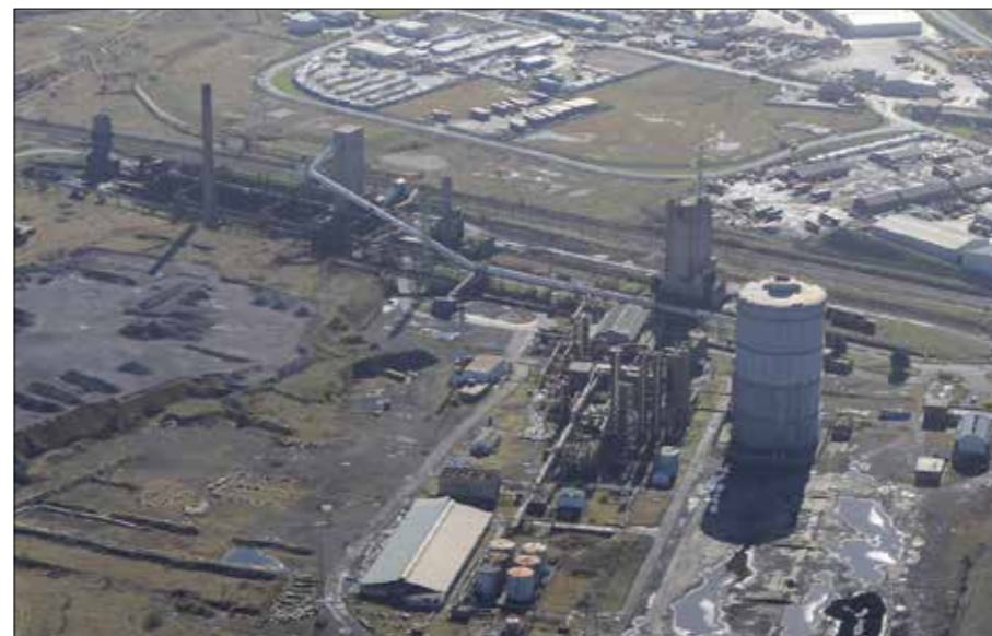
South Bank Coke Ovens
