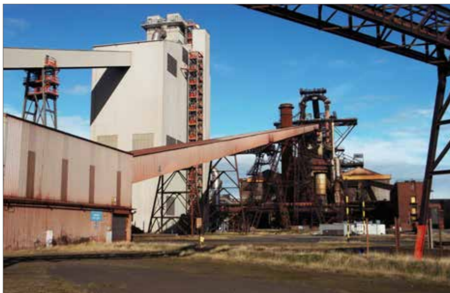
Pulverised Coal Injection Plant
