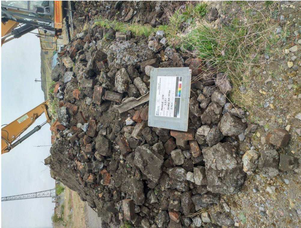
Figure PRAIRIE_AUK_TP126.3 PRAIRIE_AUK_TP126 - Spoil
