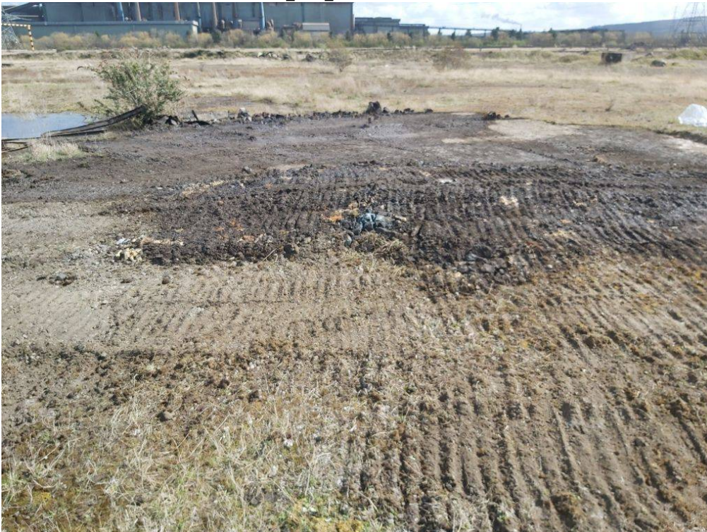
Figure PRAIRIE_AUK_TP108.4 PRAIRIE_AUK_TP108 - Reinstatement
