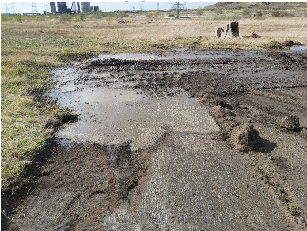
Figure PRAIRIE_AUK_TP114.4 PRAIRIE_AUK_TP114 - Reinstatement
