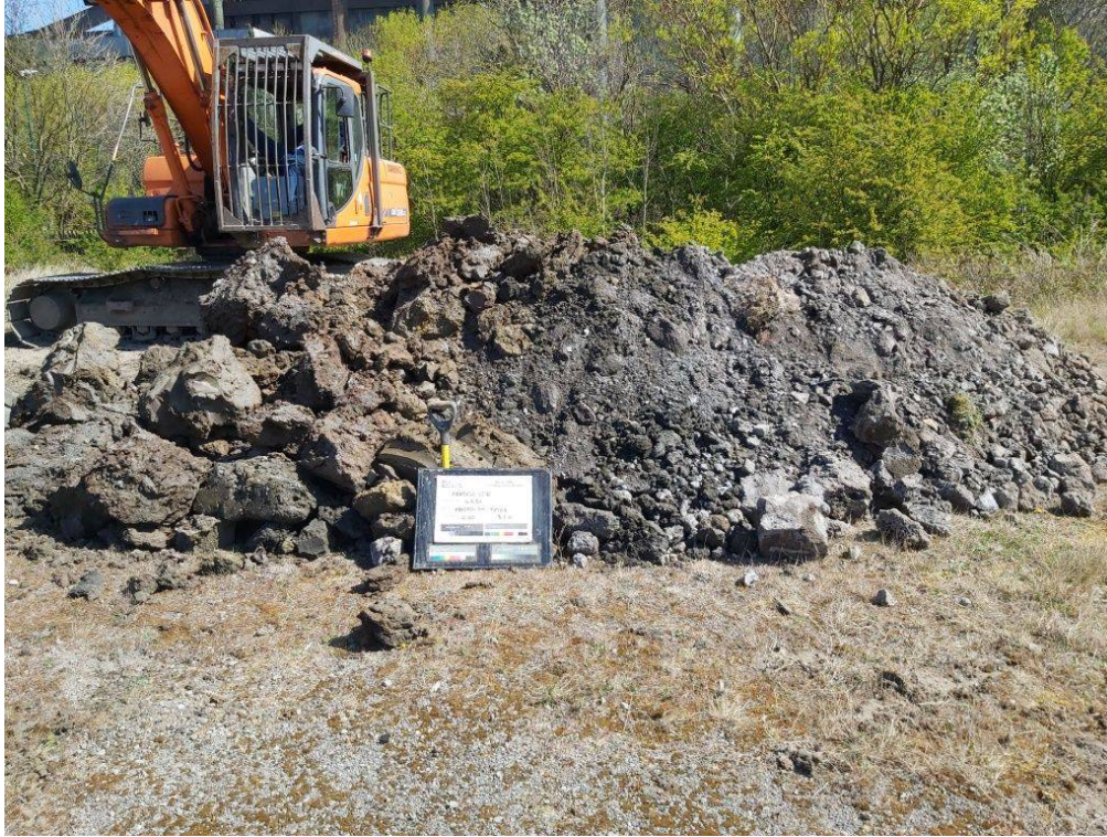
Figure PRAIRIE_AUK_TP109.3 PRAIRIE_AUK_TP109 - Spoil
