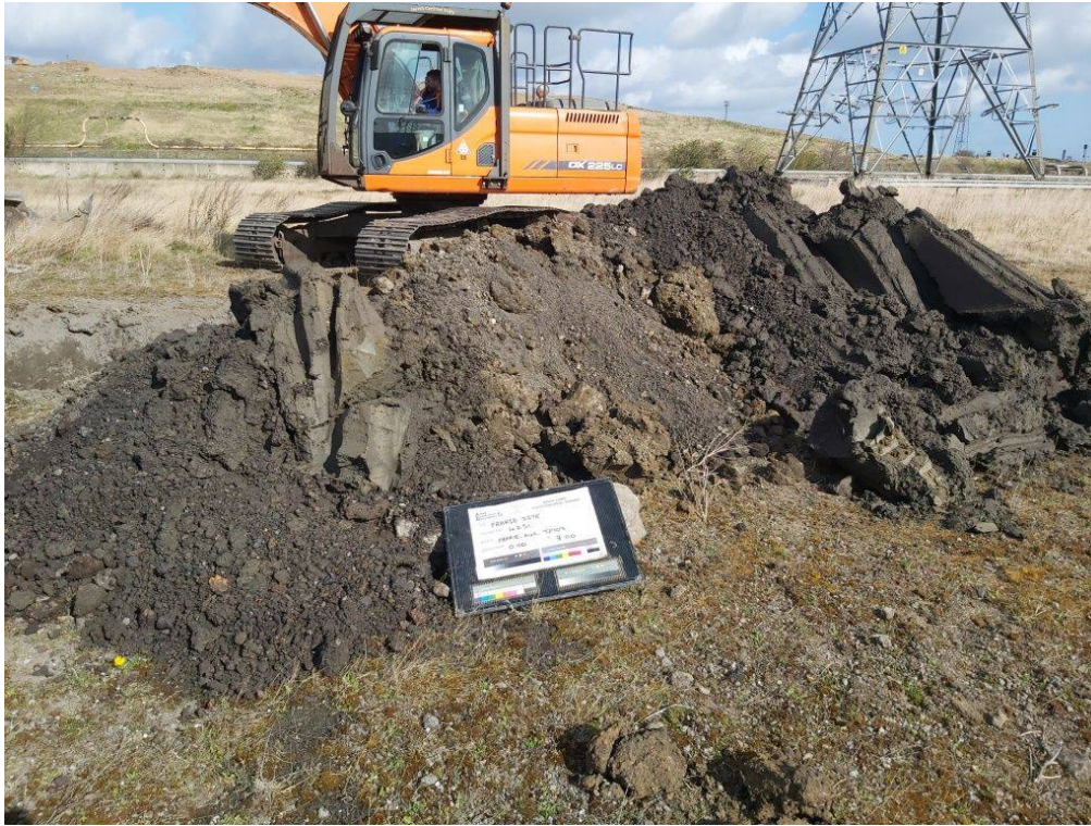
Figure PRAIRIE_AUK_TP107.3 PRAIRIE_AUK_TP107 - Spoil
