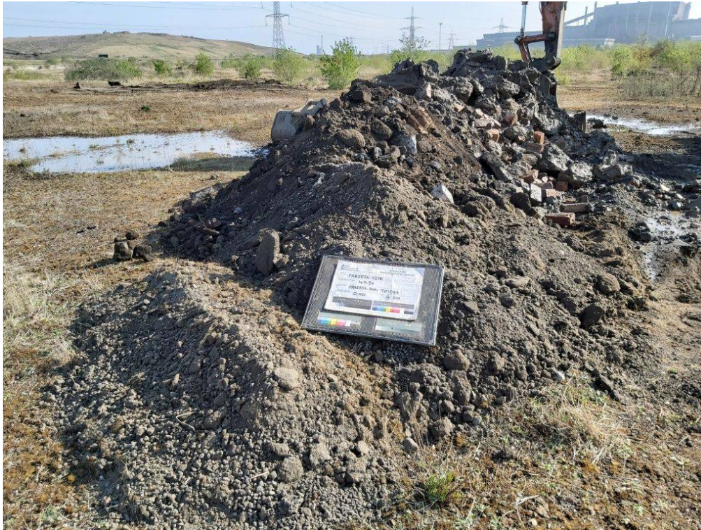
Figure PRAIRIE_AUK_TP139B.3 PRAIRIE_AUK_TP139B - Spoil
