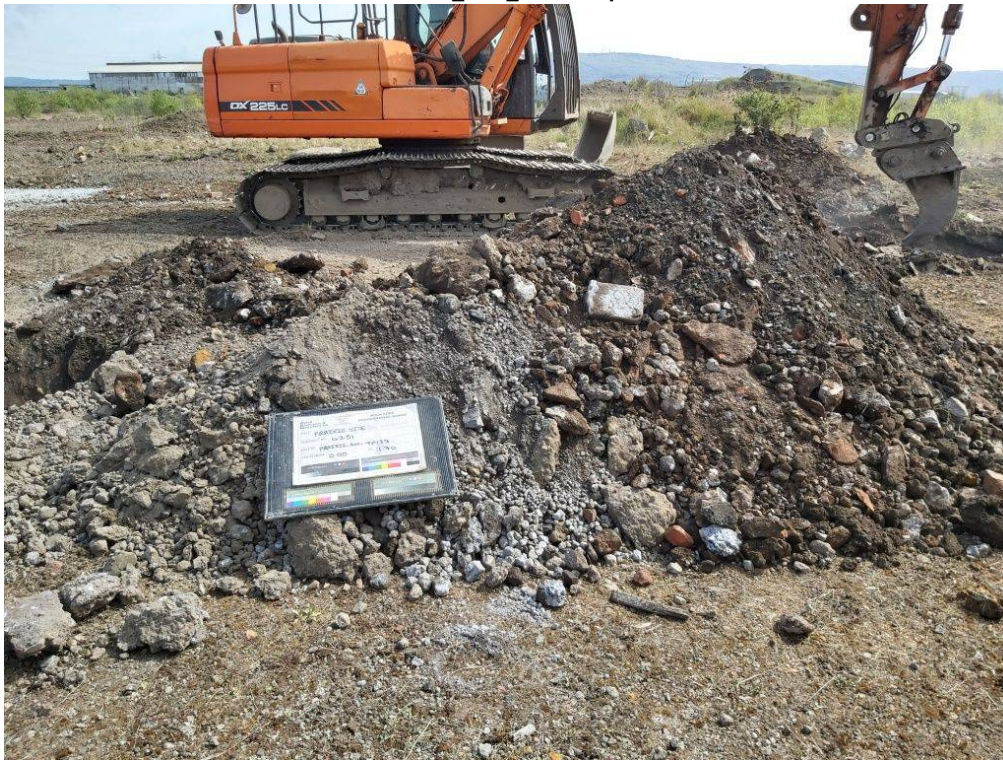
Figure PRAIRIE_AUK_TP127.3 PRAIRIE_AUK_TP127 - Spoil
