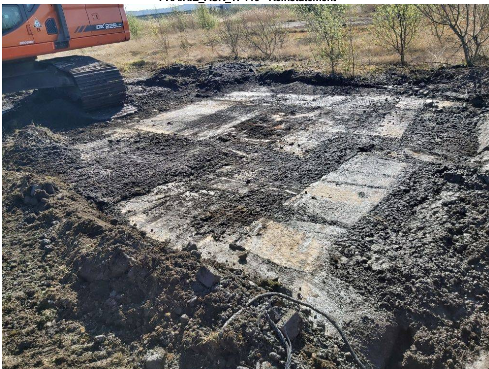
Figure PRAIRIE_AUK_TP115.4 PRAIRIE_AUK_TP115 - Reinstatement
