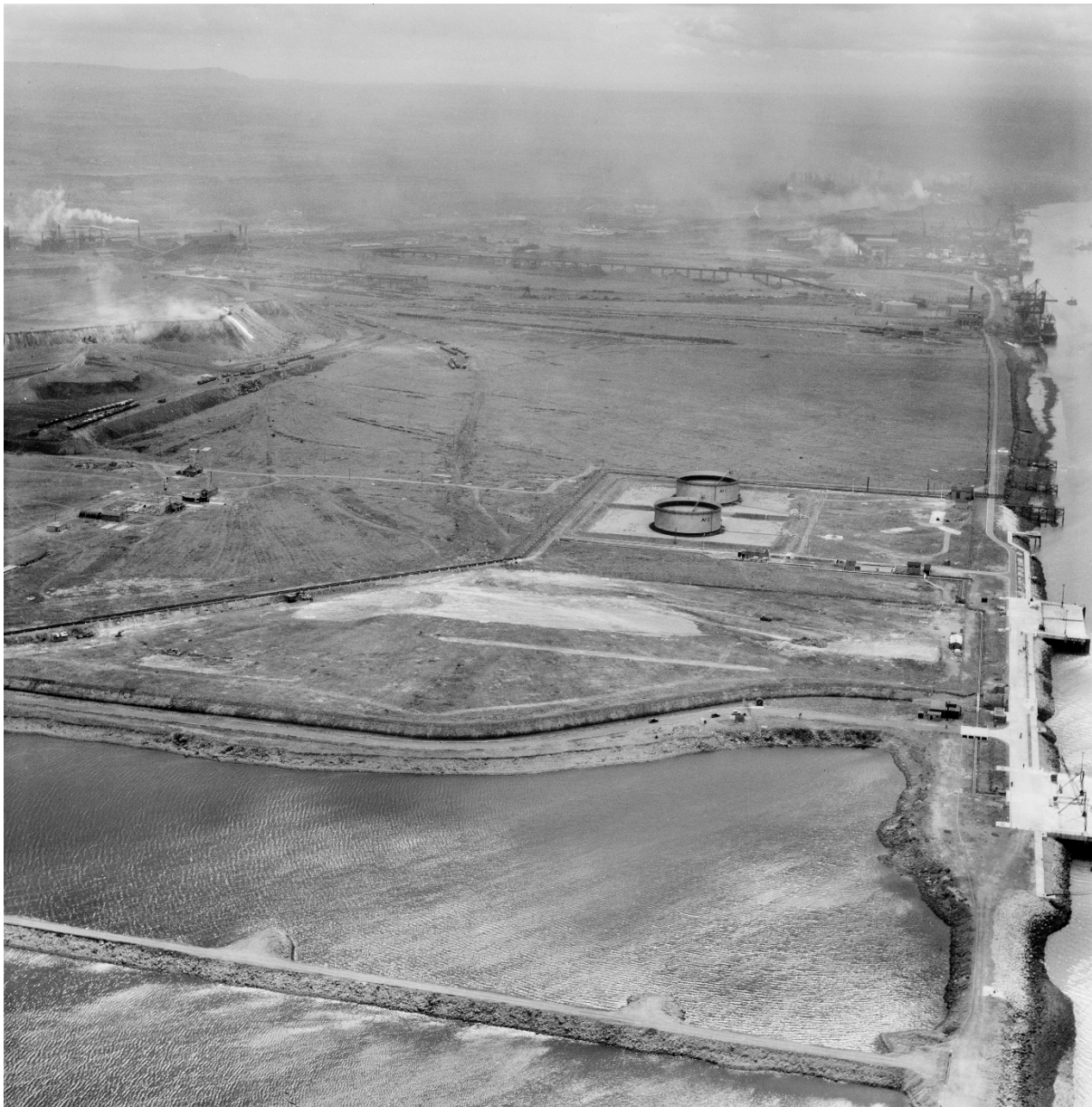
Plate 2: Looking west across the northern part of the Site with Teesport in the central right side of the photo and the South Bank Steelworks visible towards the top left. Below the steelworks, the spoil grounds are being added to with melted slag shown pouring downslope from a train. The Riverside Pumping Station is to the right, and the raised railways transporting goods to and from the wharves are visible beyond.
