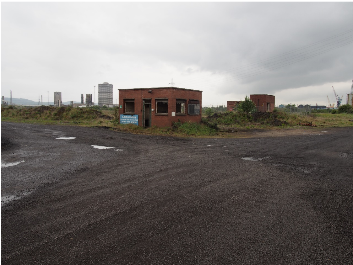
Plate 9: View south from the pumping station towards a control room, sub-station and, beyond, the gas holder and coking works in the distance
