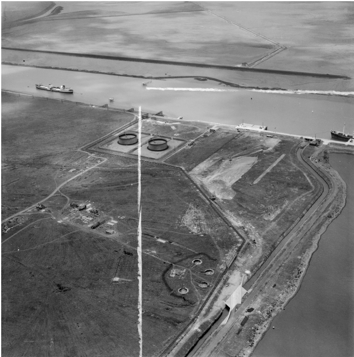
Plate 5: The HAA battery gun emplacements were still very much accessible in the 1950s, although accommodation / admin blocks are less well preserved. The bases of the WWI submarine base and later council housing can be seen immediately below the oil storage tanks.
