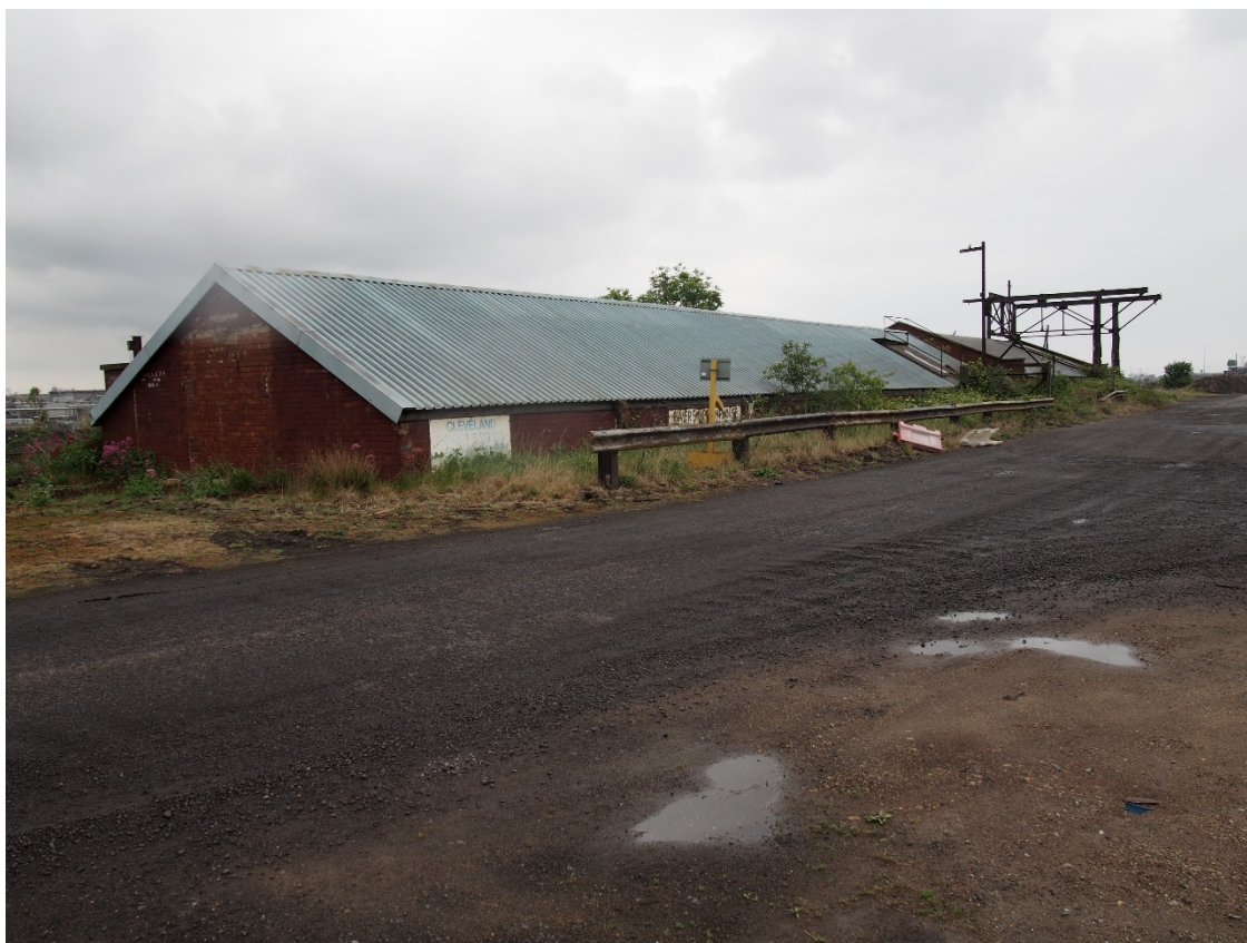
Plate 10: Riverside Pumping Station
