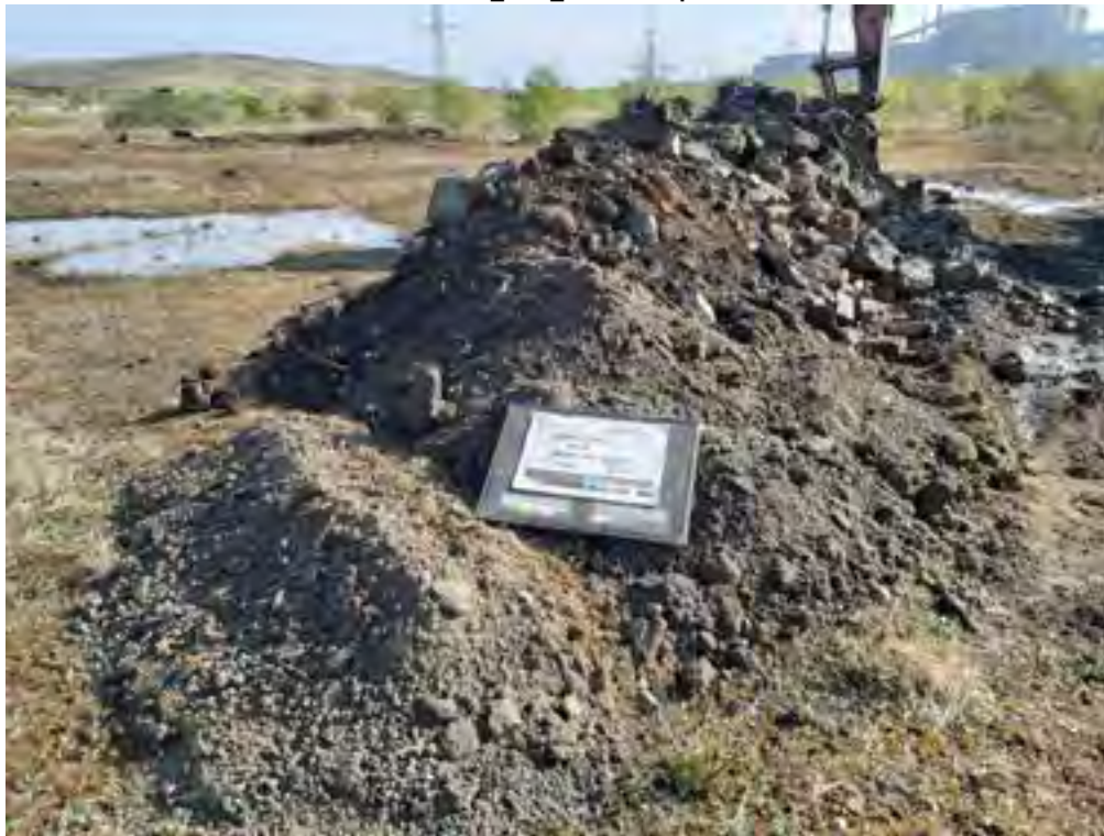
Figure PRAIRIE_AUK_TP139B.3 PRAIRIE_AUK_TP139B - Spoil
