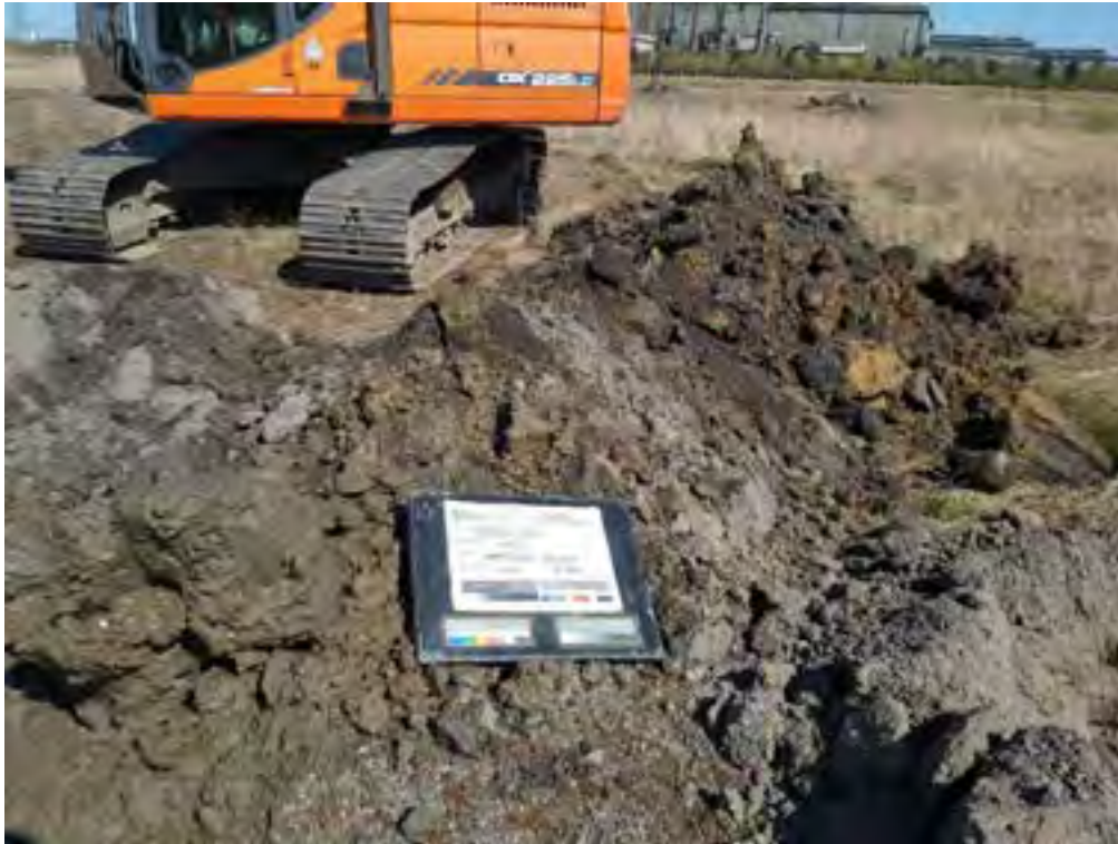
Figure PRAIRIE_AUK_TP120A.3 PRAIRIE_AUK_TP120A - Spoil
