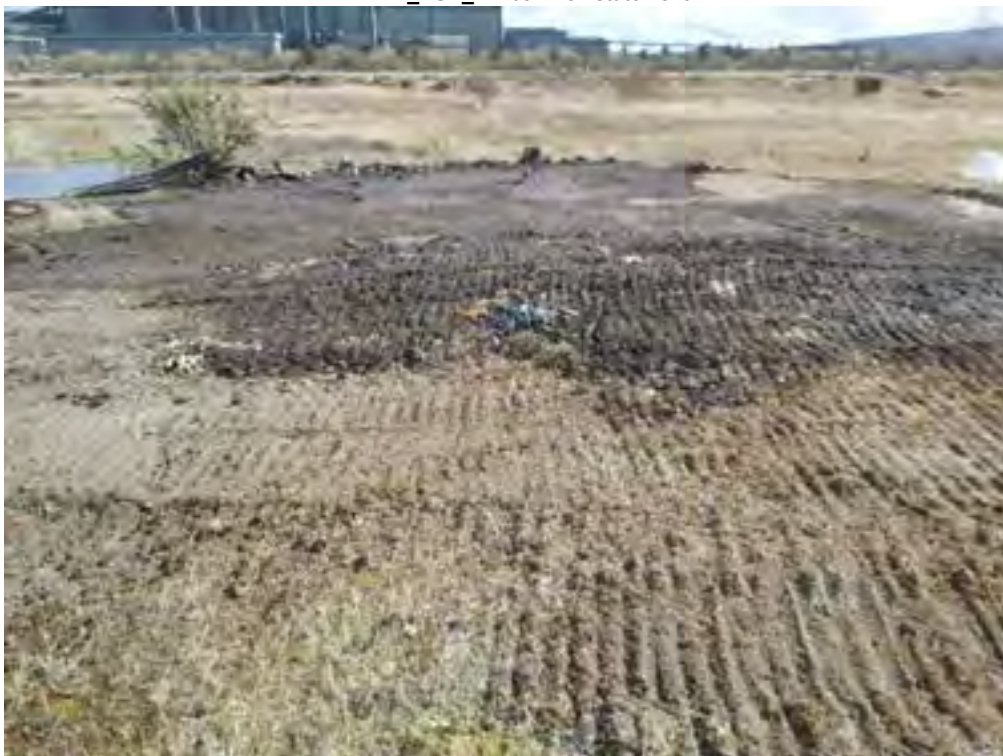
Figure PRAIRIE_AUK_TP108.4 PRAIRIE_AUK_TP108 - Reinstatement
