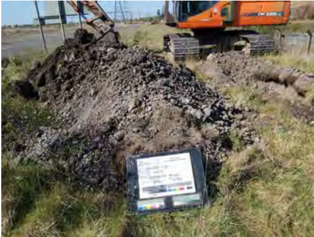
Figure PRAIRIE_AUK_TP102.3 PRAIRIE_AUK_TP102 - Spoil
