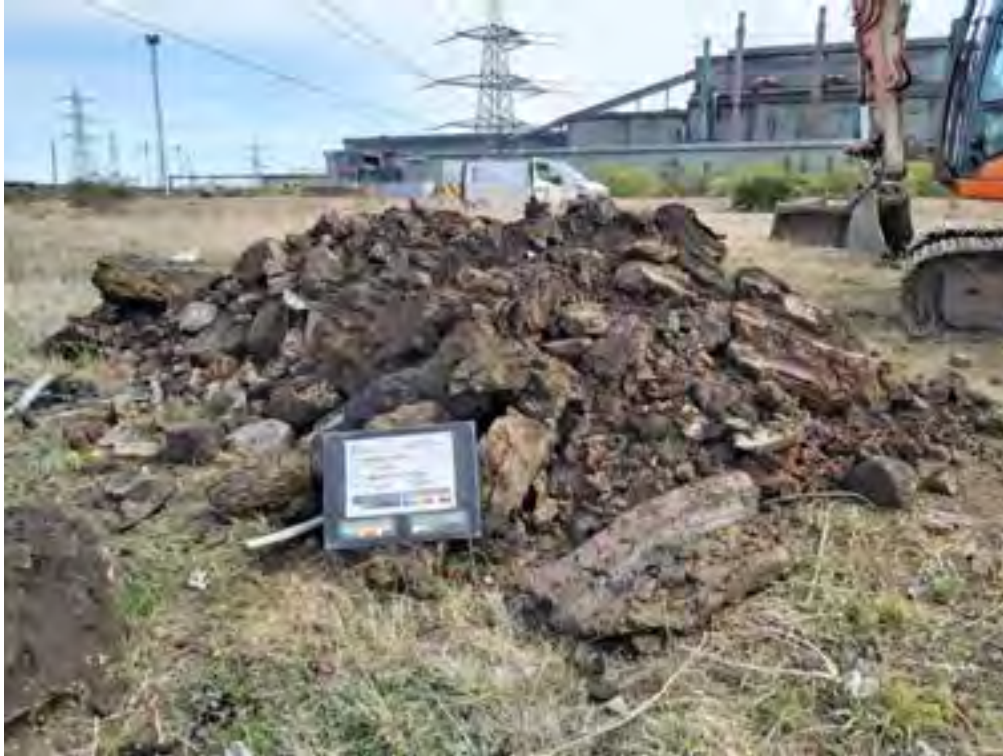
Figure PRAIRIE_AUK_TP106.3 PRAIRIE_AUK_TP106 - Spoil
