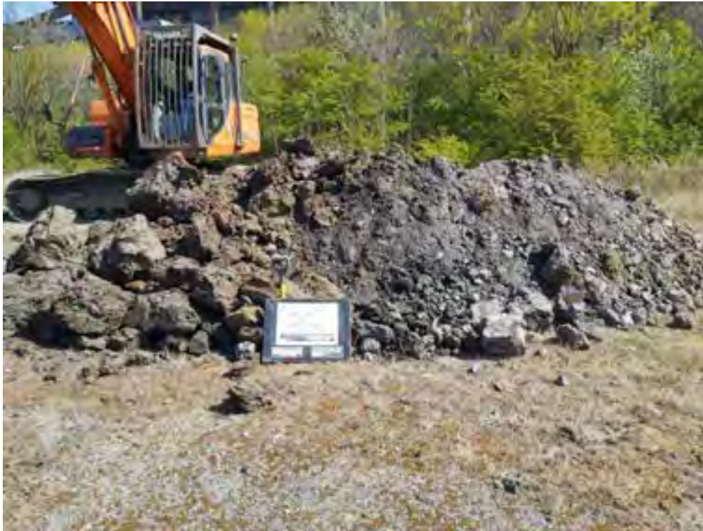
Figure PRAIRIE_AUK_TP109.3 PRAIRIE_AUK_TP109 - Spoil
