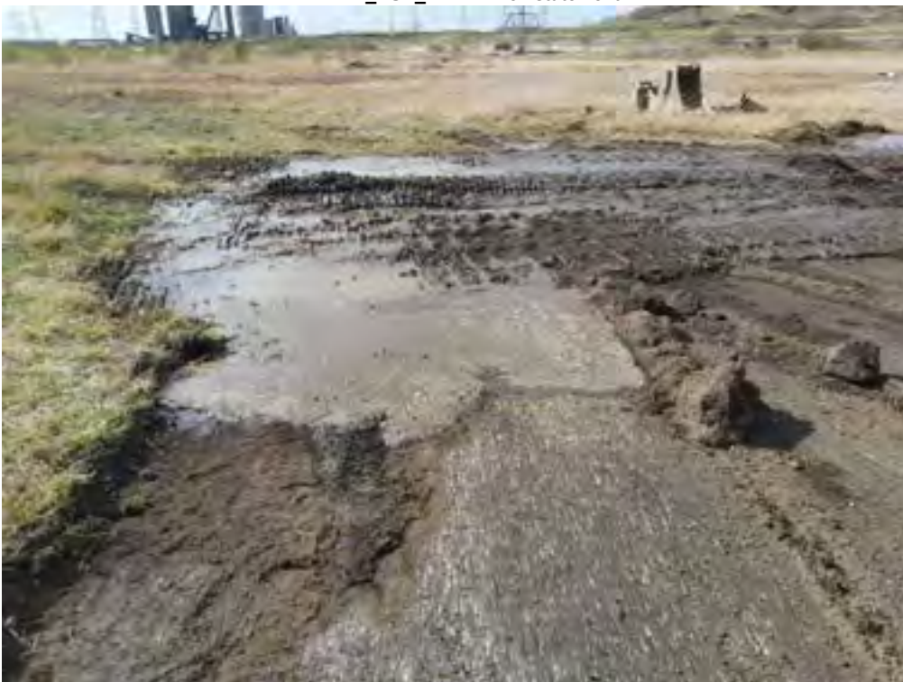
Figure PRAIRIE_AUK_TP114.4 PRAIRIE_AUK_TP114 - Reinstatement
