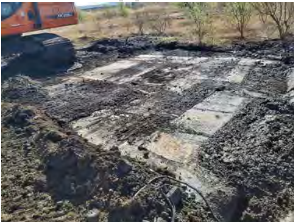
Figure PRAIRIE_AUK_TP115.4 PRAIRIE_AUK_TP115 - Reinstatement
