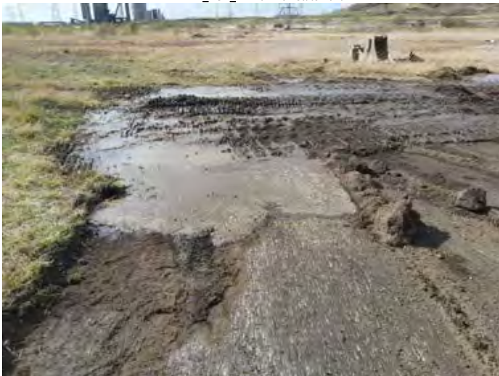
Figure PRAIRIE_AUK_TP113.4 PRAIRIE_AUK_TP113 - Reinstatement
