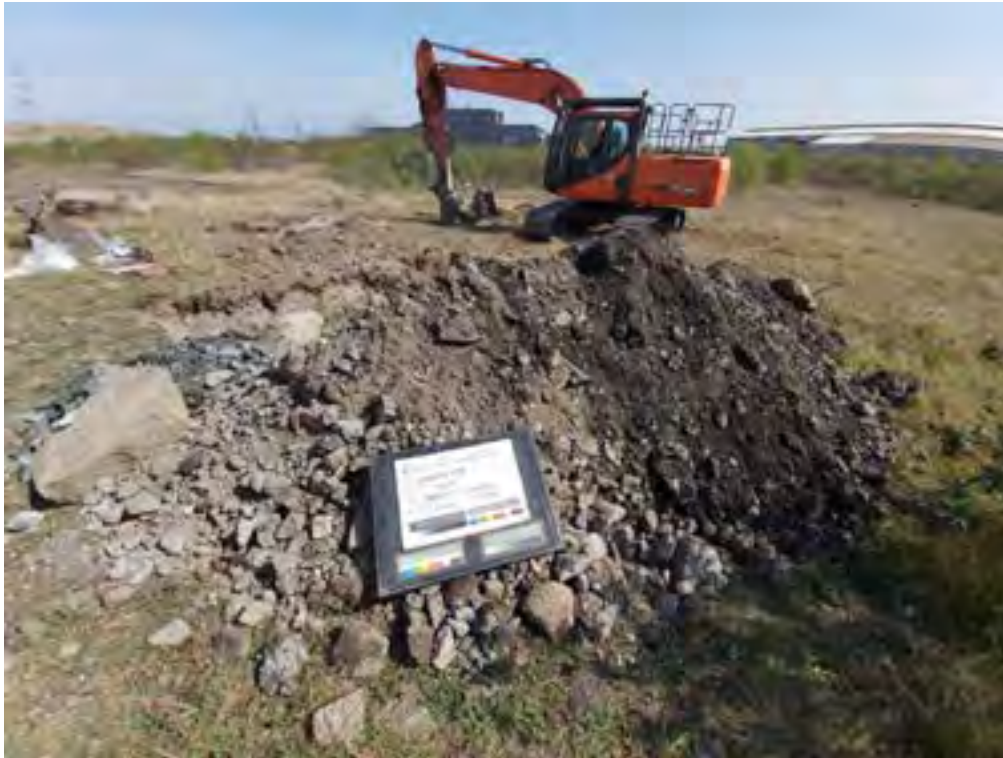
Figure PRAIRIE_AUK_TP148A.3 PRAIRIE_AUK_TP148A - Spoil
