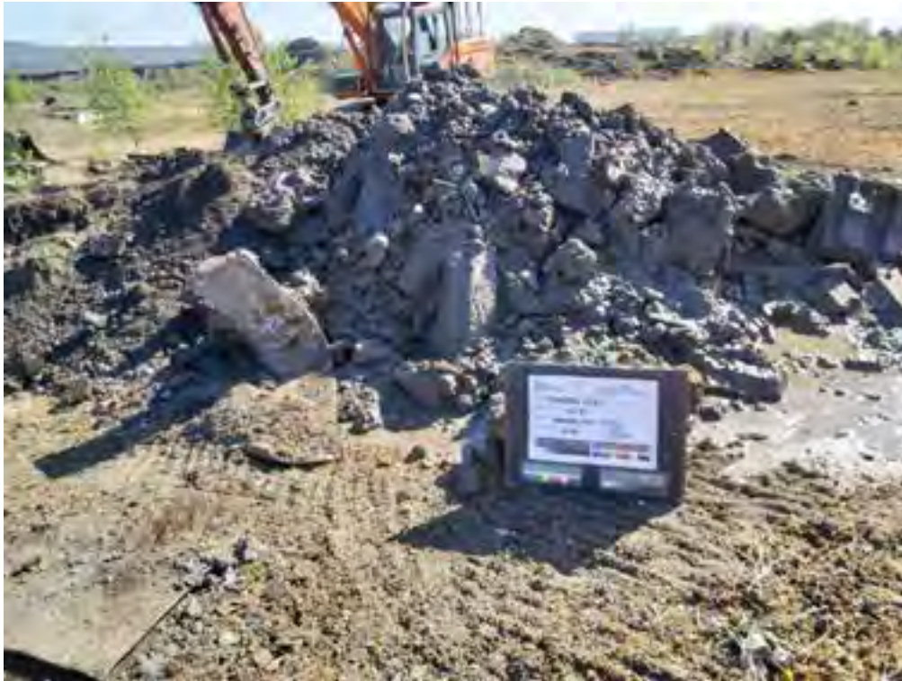
Figure PRAIRIE_AUK_TP137.7 PRAIRIE_AUK_TP137 - Spoil
