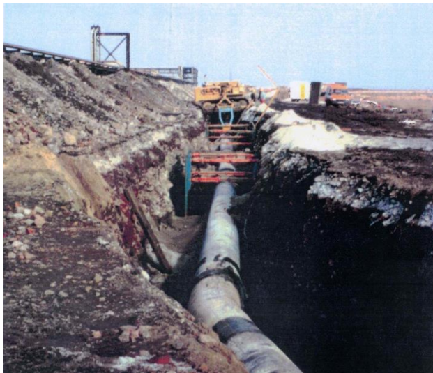
Construction Images of the 36" pipeline routing through South Tees industrial sites
