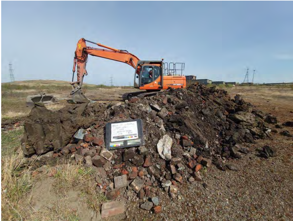
Figure PRAIRIE_AUK_TP146C.3 PRAIRIE_AUK_TP146C - Spoil
