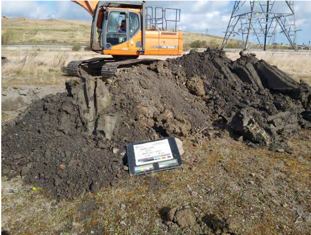
Figure PRAIRIE_AUK_TP107.3 PRAIRIE_AUK_TP107 - Spoil
