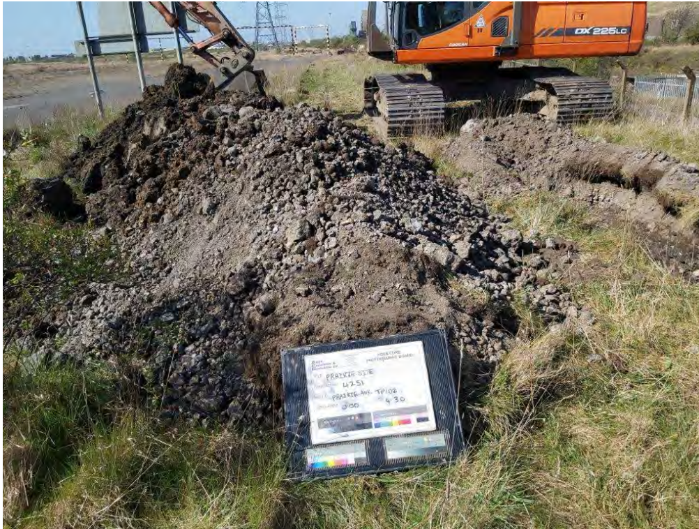
Figure PRAIRIE_AUK_TP102.3 PRAIRIE_AUK_TP102 - Spoil
