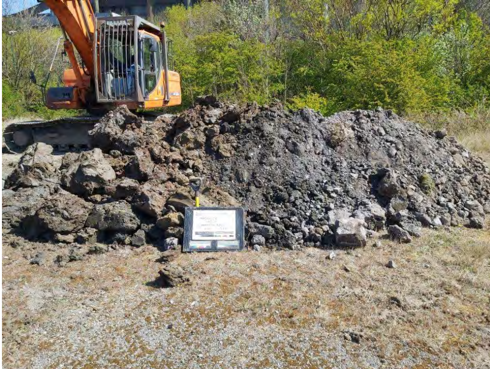
Figure PRAIRIE_AUK_TP109.3 PRAIRIE_AUK_TP109 - Spoil
