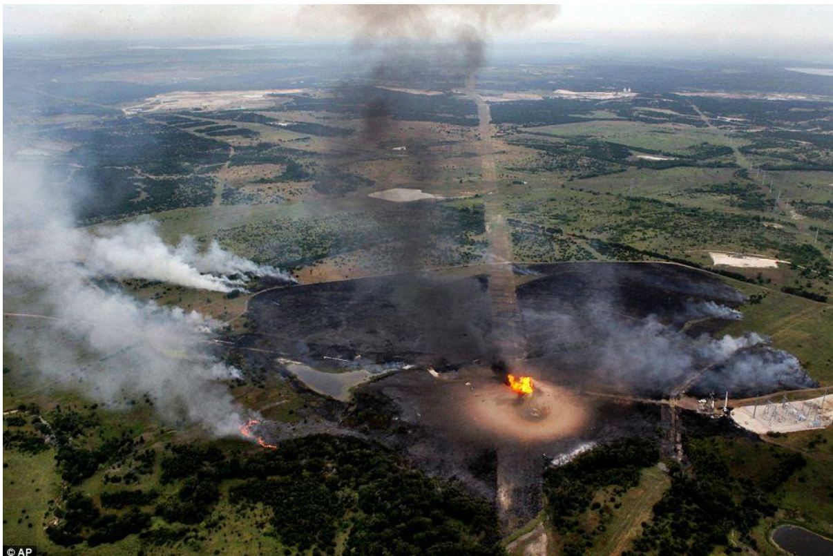
36" Gas Pipeline Explosion, North Texas June 7, 2010
