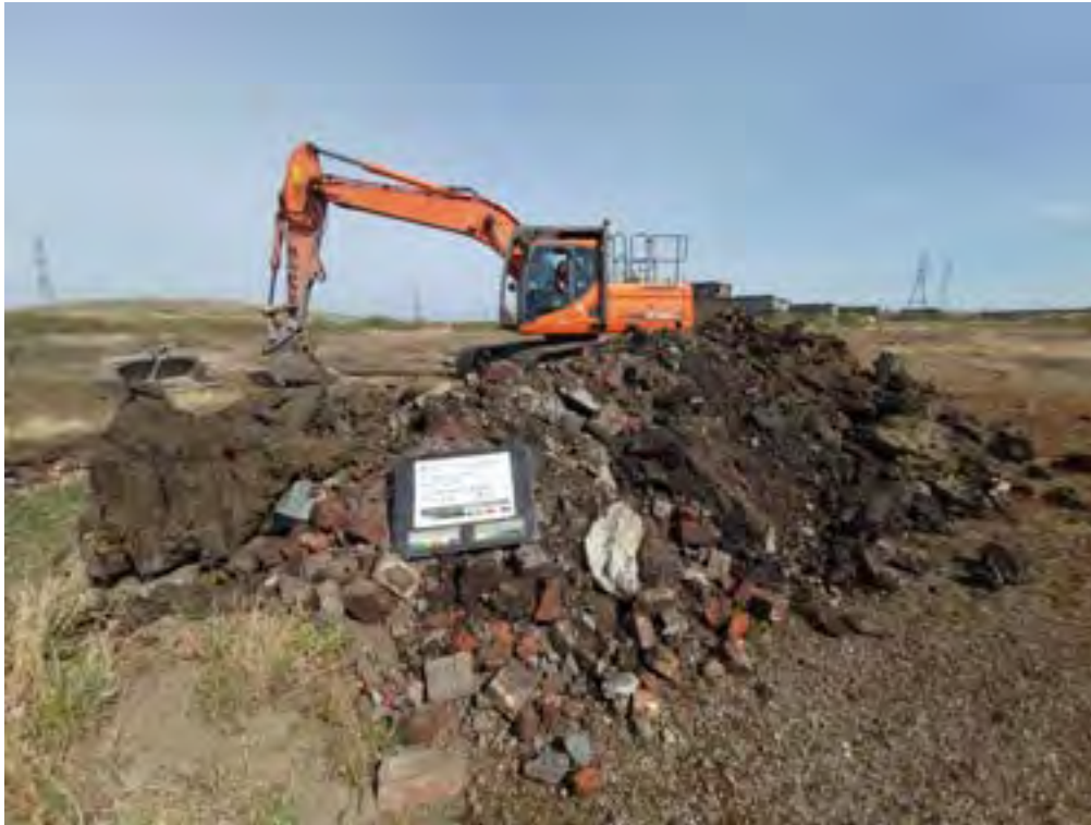
Figure PRAIRIE_AUK_TP146C.3 PRAIRIE_AUK_TP146C - Spoil
