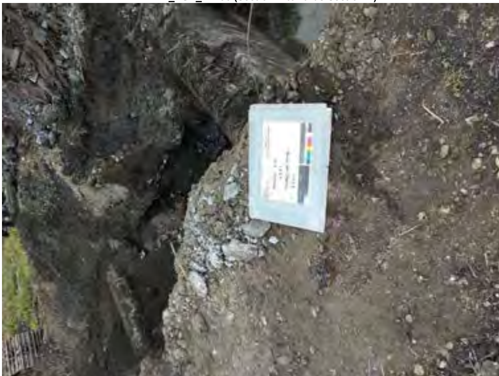
Figure PRAIRIE_AUK_TP196B.4 PRAIRIE_AUK_TP196 (Section B towards Section A)
