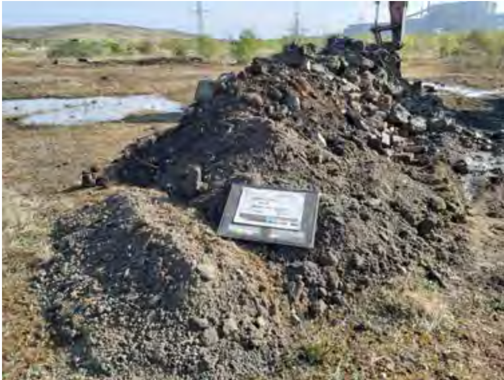
Figure PRAIRIE_AUK_TP139B.3 PRAIRIE_AUK_TP139B - Spoil
