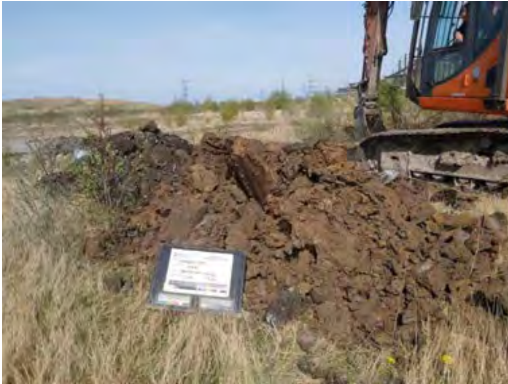
Figure PRAIRIE_AUK_TP156A.3 PRAIRIE_AUK_TP156A - Spoil
