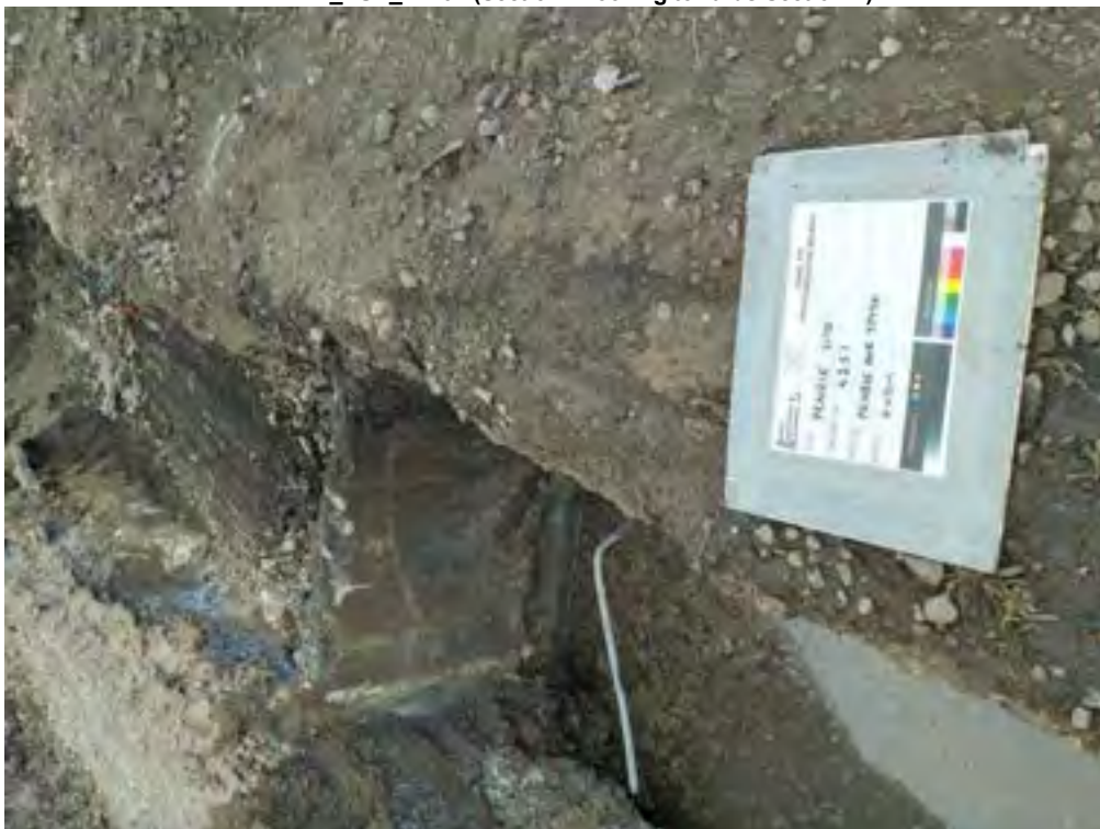
Figure PRAIRIE_AUK_TP194C.2 PRAIRIE_AUK_TP194 (Section B looking towards Section C)
