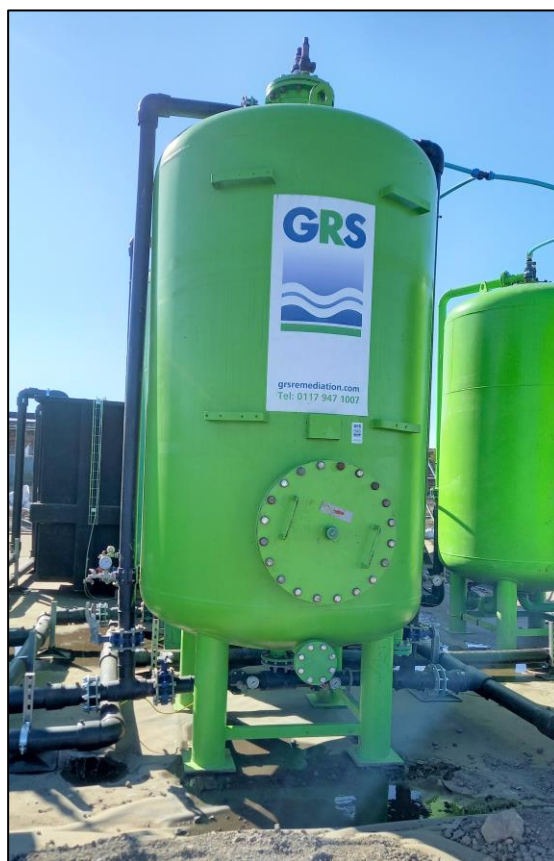
Figure 10. BI50 carbon vessel (GAC)
