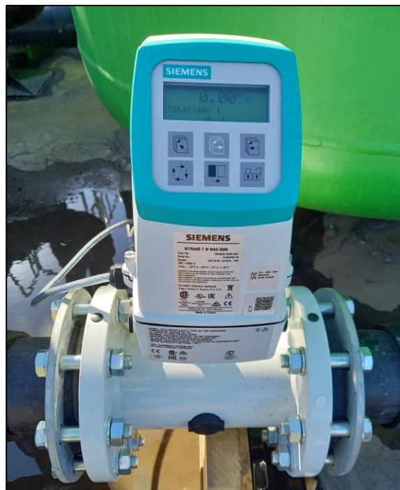
Figure 14. Electromagnetic flowmeter
