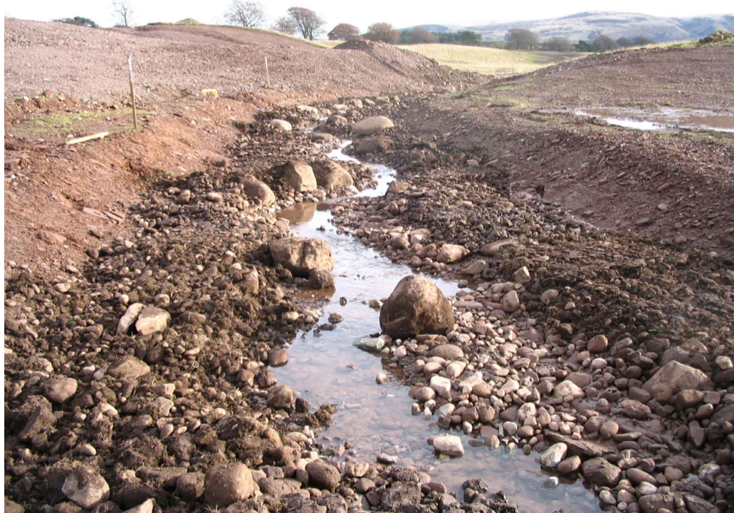
EXAMPLE OF LOW FLOW CHANNEL GRANULAR SUBSTRATE
