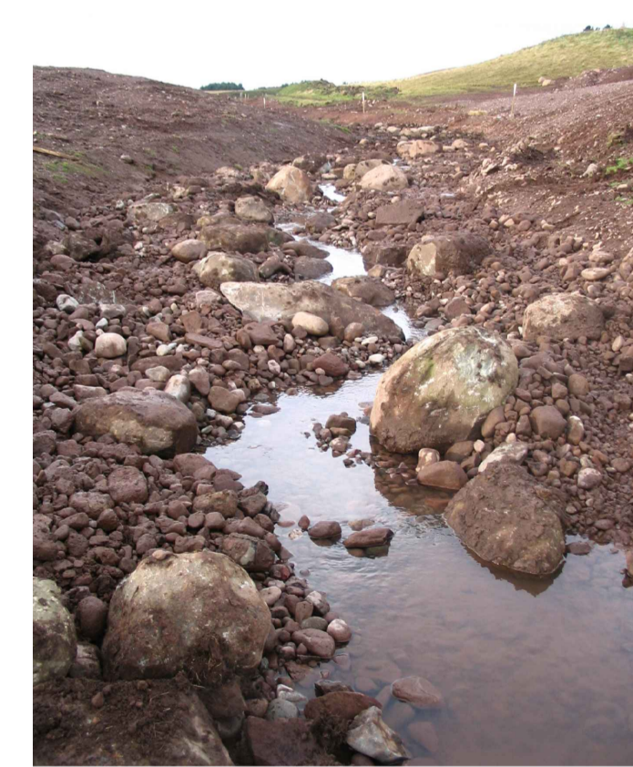
EXAMPLE OF LOW FLOW CHANNEL GRANULAR SUBSTRATE
