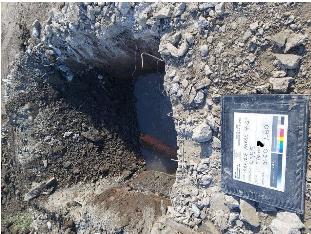
Figure S3_TPA_TP107.2 S3_TPA_TP107
