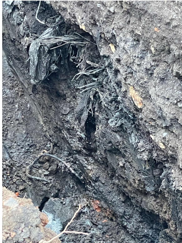
Plate 1: Potential hydrocarbon impact identified within SHO-TS1_AUK_TP102
