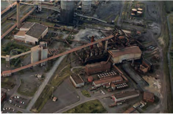
Redcar Blast Furnace
