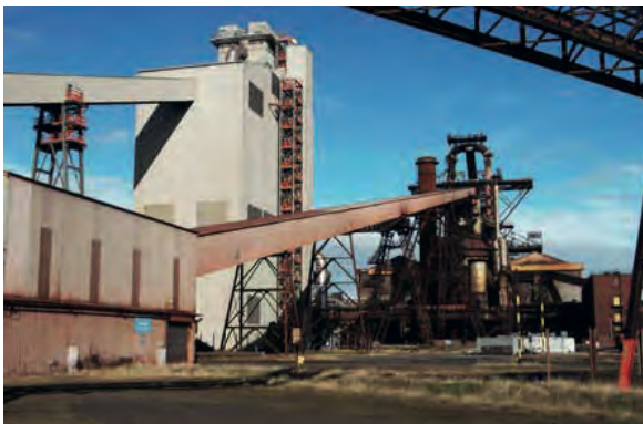
Pulverised Coal Injection Plant at Redcar Blast Furnace
