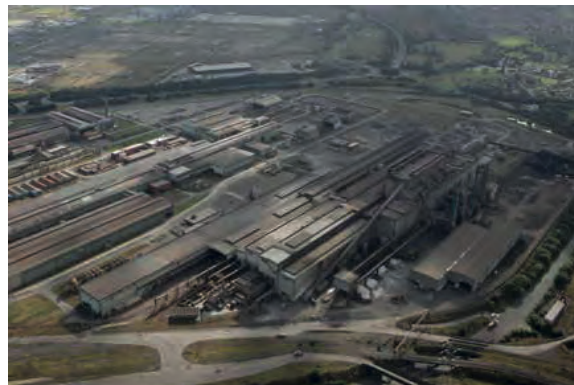
Lackenby Steelmaking Complex
