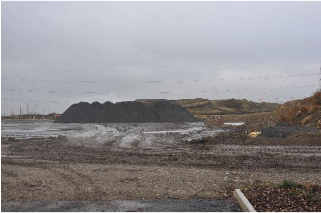
Plate 3: Eastern boundary of site, adjoining adjacent plot. Photo from 2023 site visit
