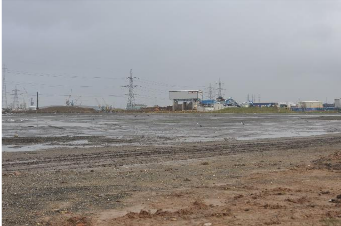
Plate 1: View north across site. Photo from 2023 site visit
